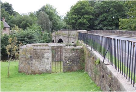
Pound on North East Side of Wennington Bridge
